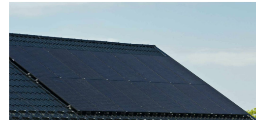
Solar panels with black background and black frames, setout in a uniform manner and mounted flat to the roof.
