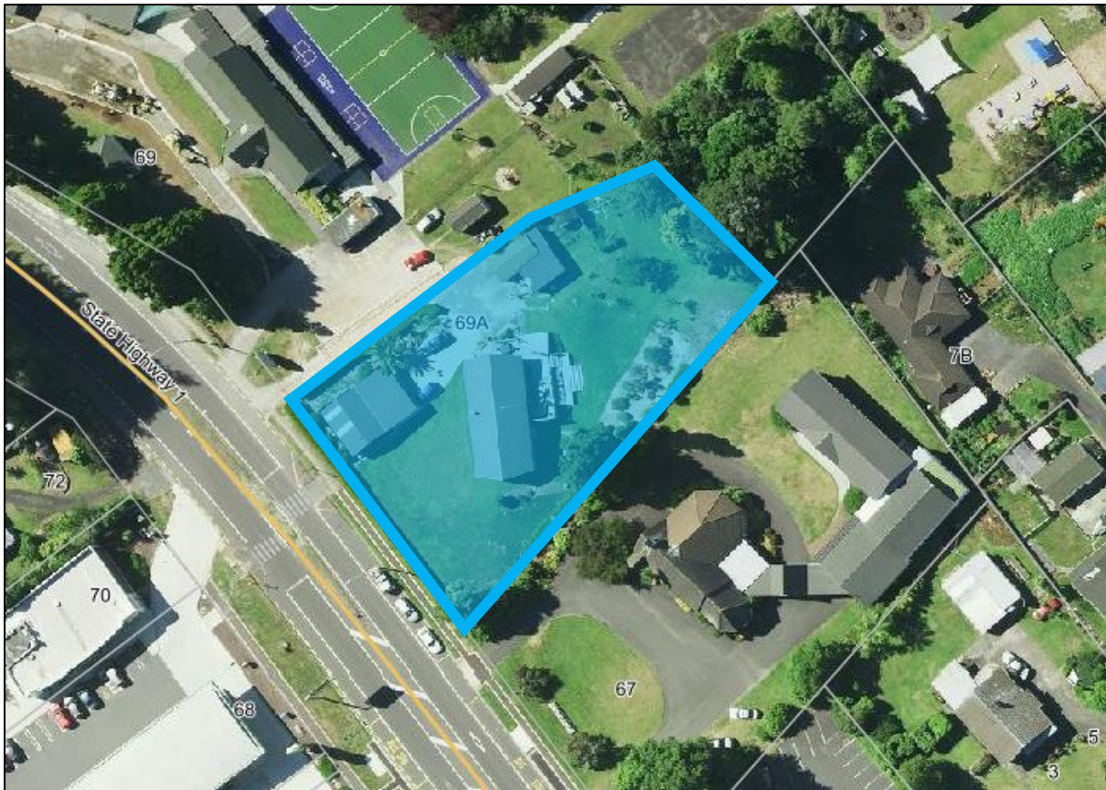
Figure 1: Aerial Photograph of Subject Site
